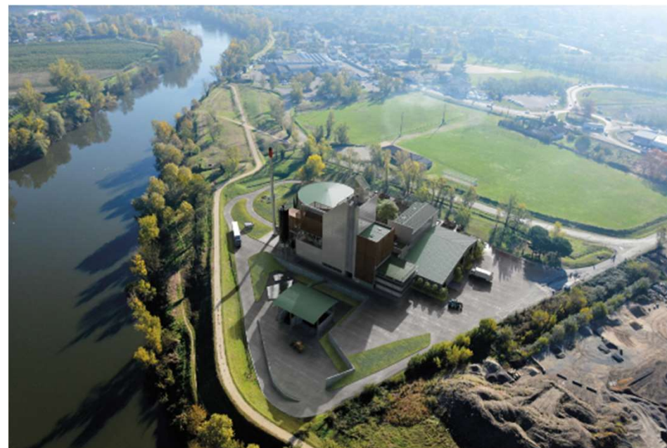
Ramping up of Mo'Uve (Montauban - France)
