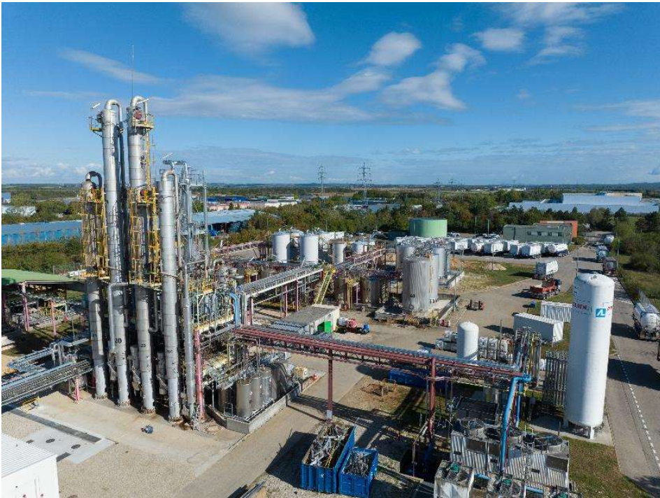
Solvent regeneration and chemical purification (Speichim Processing - France)
