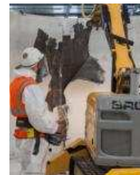
Asbestos removal at Le Havre
