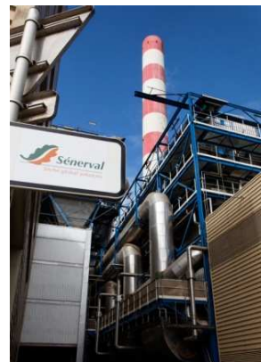
Expansion of heating network at Strasbourg-Sénerval
