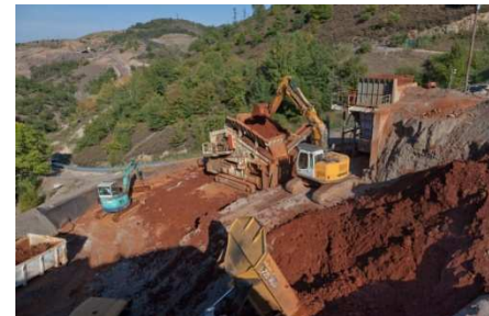
Heavy metal decontamination at Viviez
