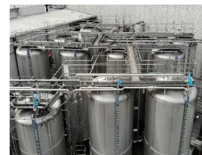
Mecomer: hazardous waste sorting and grouping
