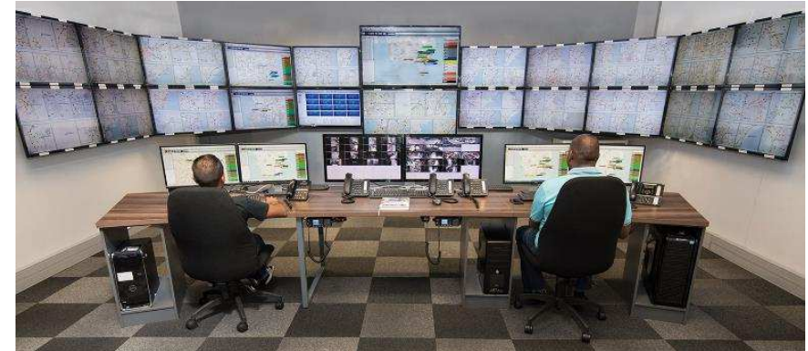
Operational control room
