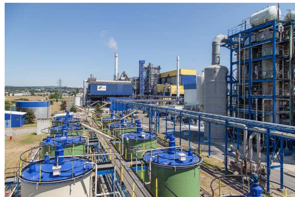
Installations de Salaise-sur-Sanne
