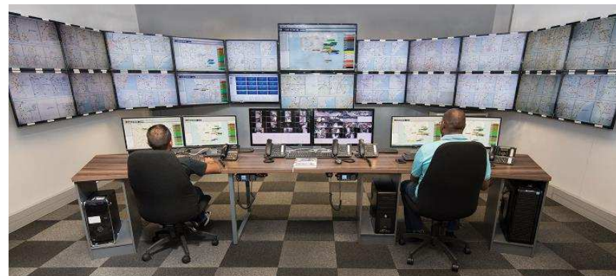
Operational control room
