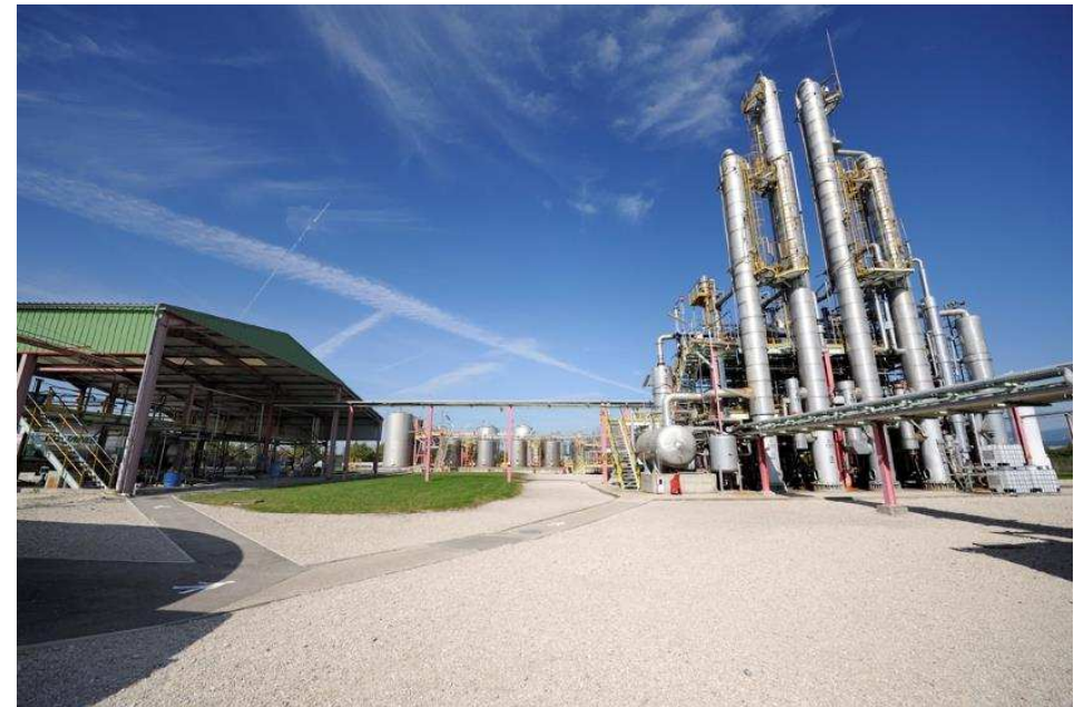
Chemical purification – Speichim Processing
