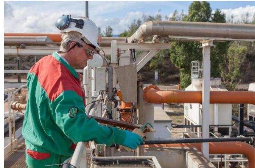
Delegated management of waste treatment facilities
