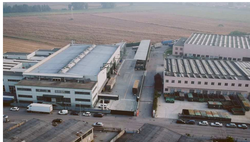
Extension of the capacities of the San Giuliano Milanese facility, Mecomer, Italy
