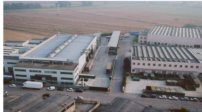
Extension of the capacities of the San Giuliano Milanese facility, Mecomer, Italy
