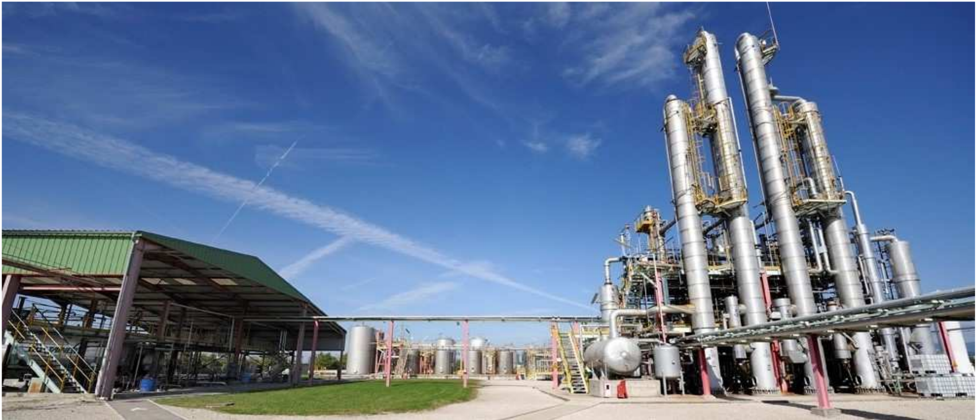
Speichim Processing, St Vulbas, France
