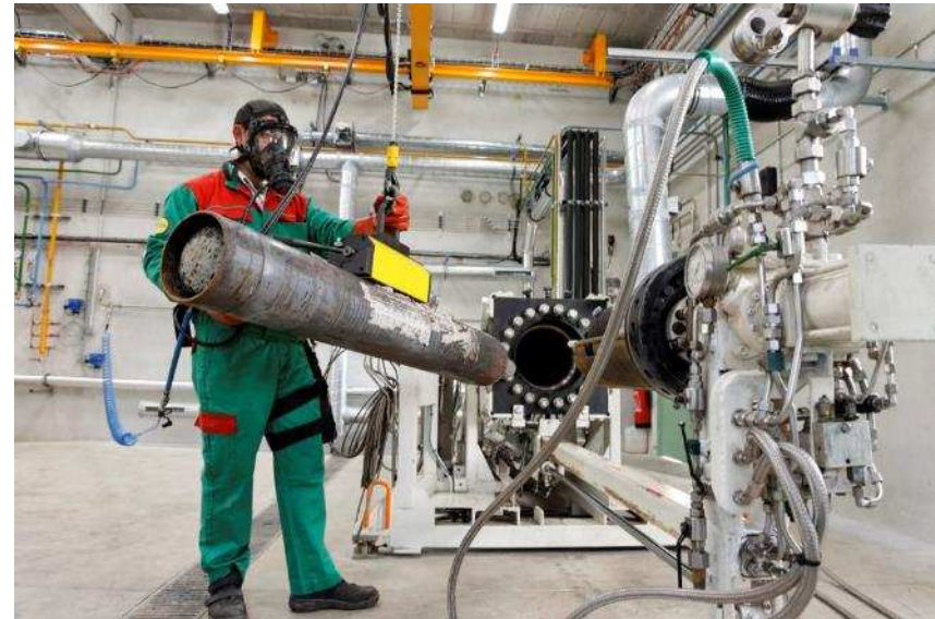
Industrial gas treatment Saint-Vulbas site, France
