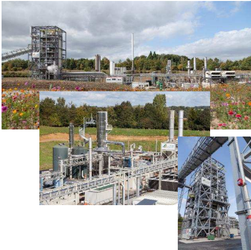
Energy recovery facility Changé site, France
