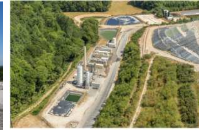
Energy recovery La-Croix-Irtelle (Morbihan)
