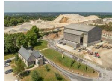
Household and Economic activities waste sorting center HW transfer platform Nivallac (Morbihan)
