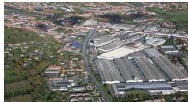
The Arc International industrial site
